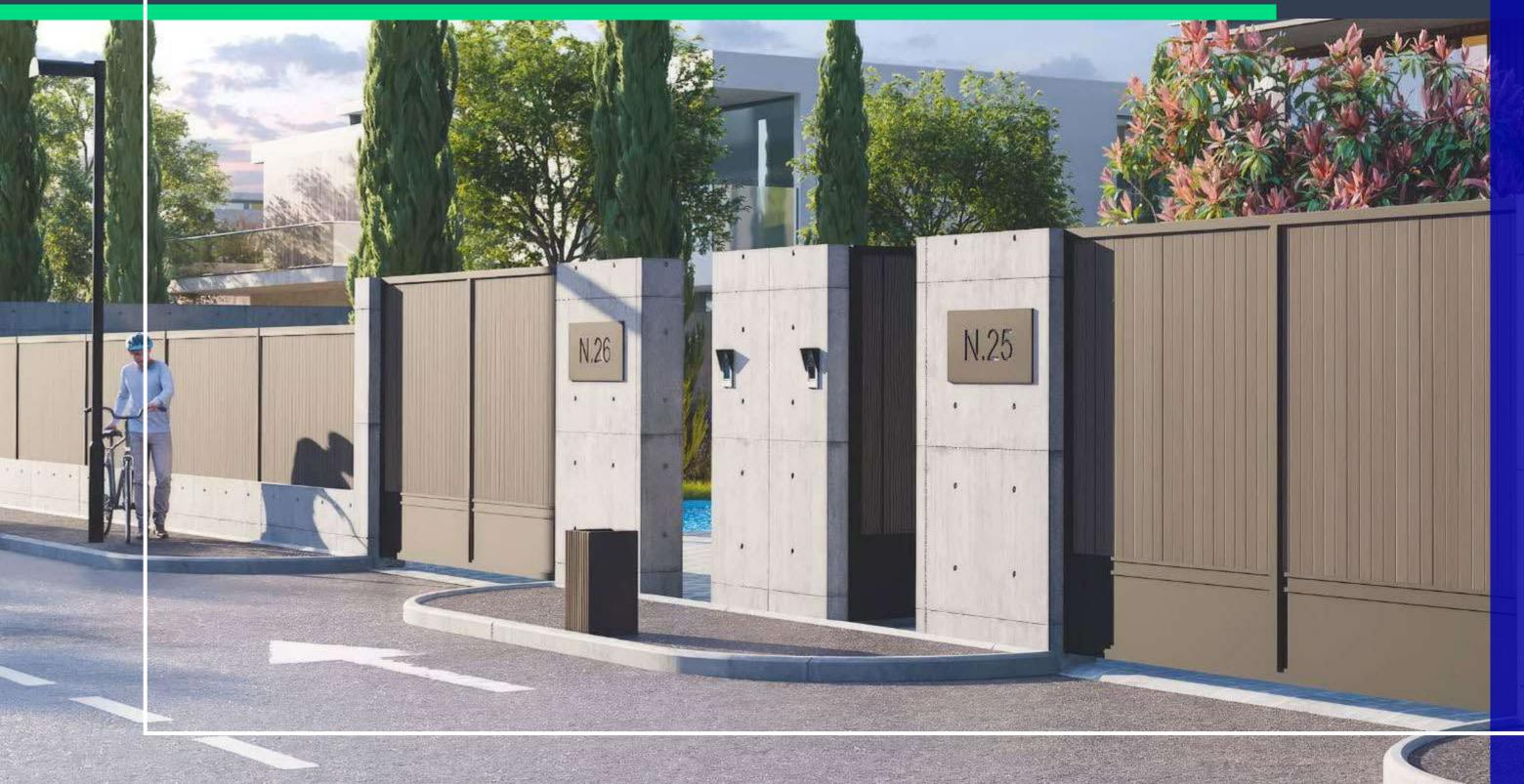
The plot will feature a fence of up to 1.8 meters in height at the entrance, constructed using a combination of concrete plinth and decking material.
